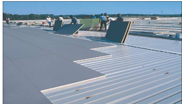
Figure 9 TPO roofing installing process, image courtesy www.summitroofing.info
