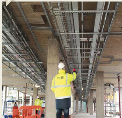
Workers are doing the final steps of the installation process
