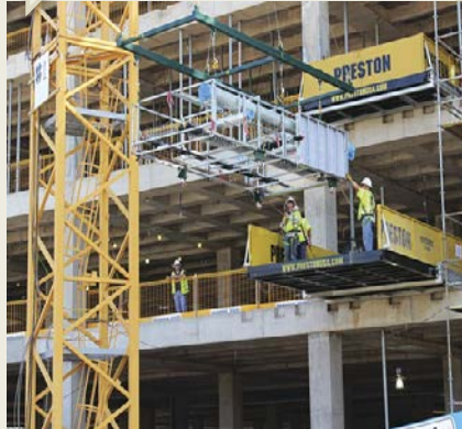
Manpower is used to assist the placing process
