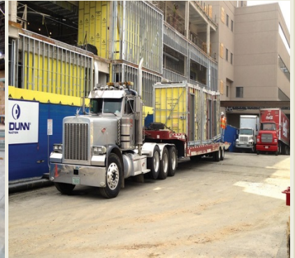
The MEP system compenets are dilivered to the site.
