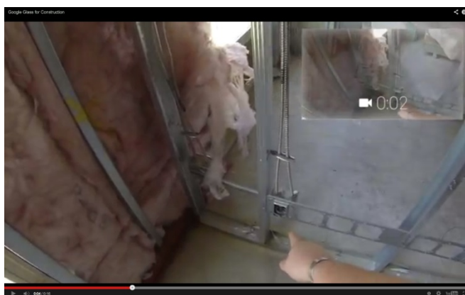
Figure 49 Todd Wynne using live webcam to communicate with the project architect. Image courtesy of www.bdcnetwork.com
