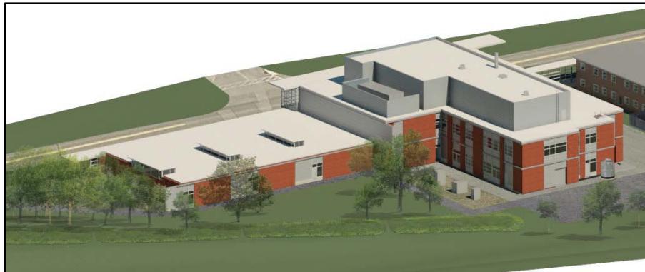
Figure 7 an aerial view of Educational Activities Building. Image courtesy of BCJ
